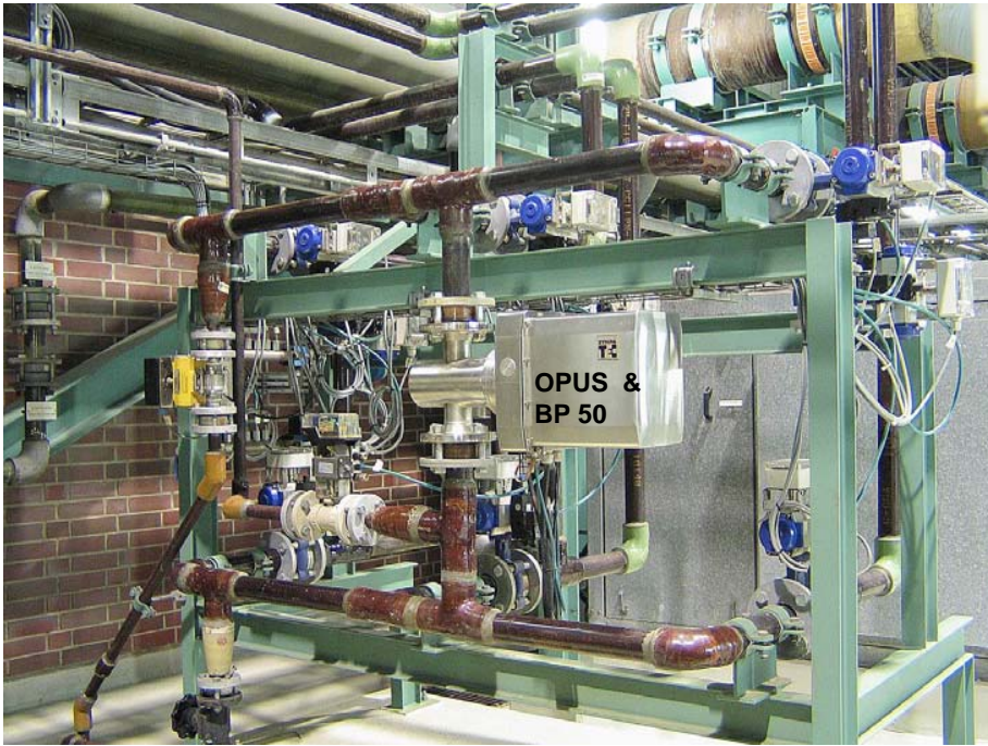
Fig. 11: The OPUS Probe installed in a complex sampling station using a bypass adapter with 50 mm Ø
